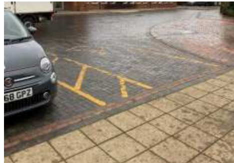
Repainting parking areas
