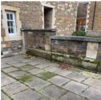
School House Ramp area
